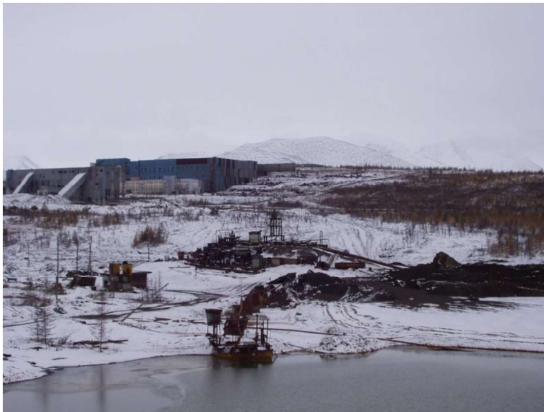
Fig. 1 General view of the enterprise
